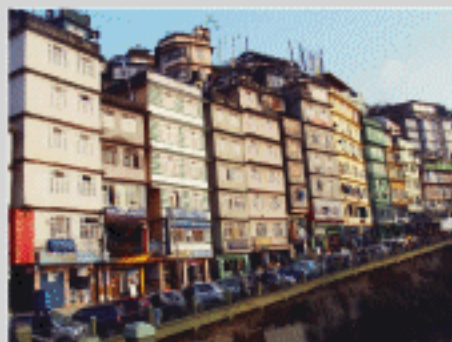
Eight plus storey buildings in Gangtok built on apparently non-ductile beam column frames with little or no breathing space in between calls for stringent norms for construction regulation and policy frame work, failing which debris demolition cost would surpass actual reconstruction demands.
